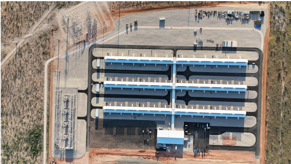
Black Pearl Phase I, the first 150 MW of the 300 MW site, is energized and hashing.
