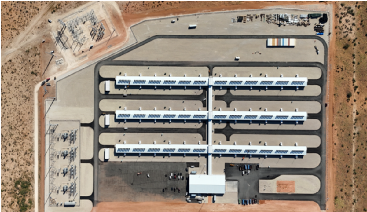
Black Pearl Phase I, the first 150 MW of the 300 MW site, is steadily ramping production as new rigs continue to be delivered.
