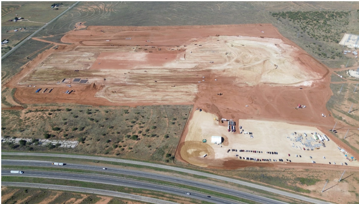
Construction underway at Barber Lake.
