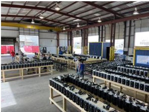
Odessa Data Center Staging Area
