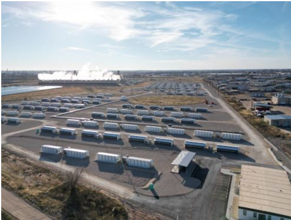
Odessa Data Center Area B & C
