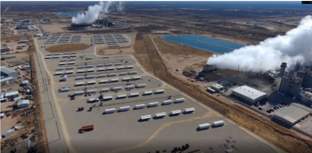
Odessa Data Center Area B & C
