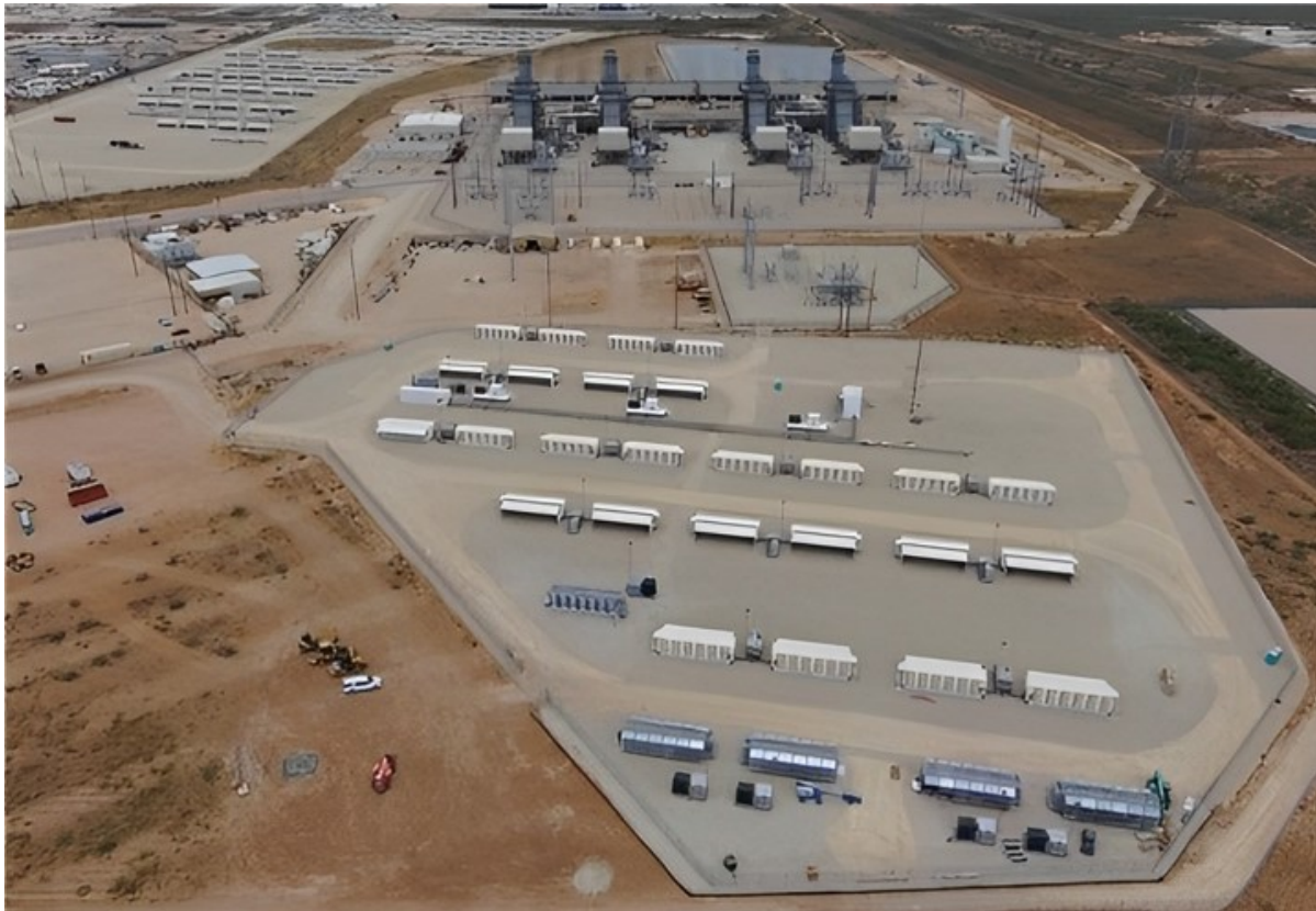
Our Odessa Data Center, with recently deployed infrastructure in the foreground
