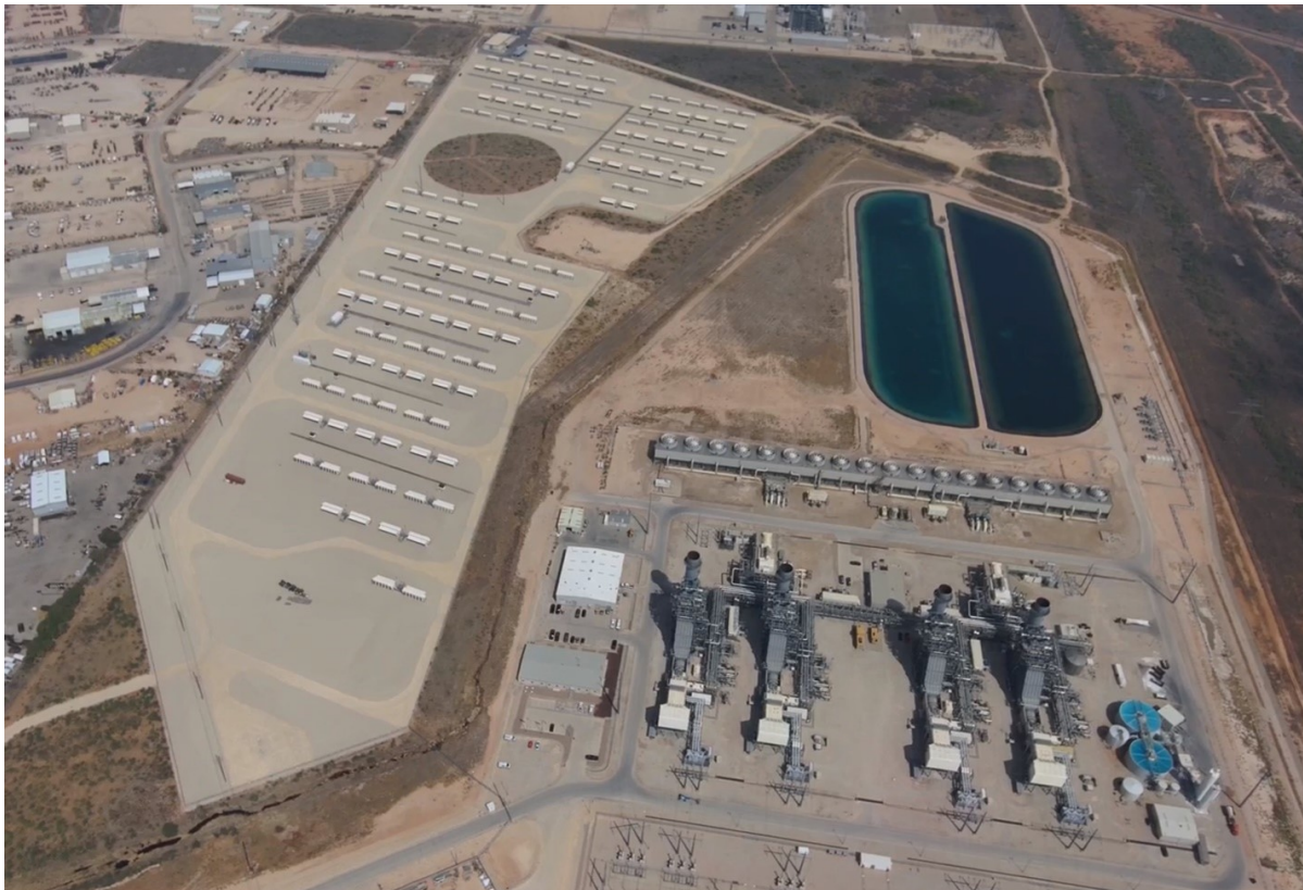
Cipher Mining's Odessa Facility
