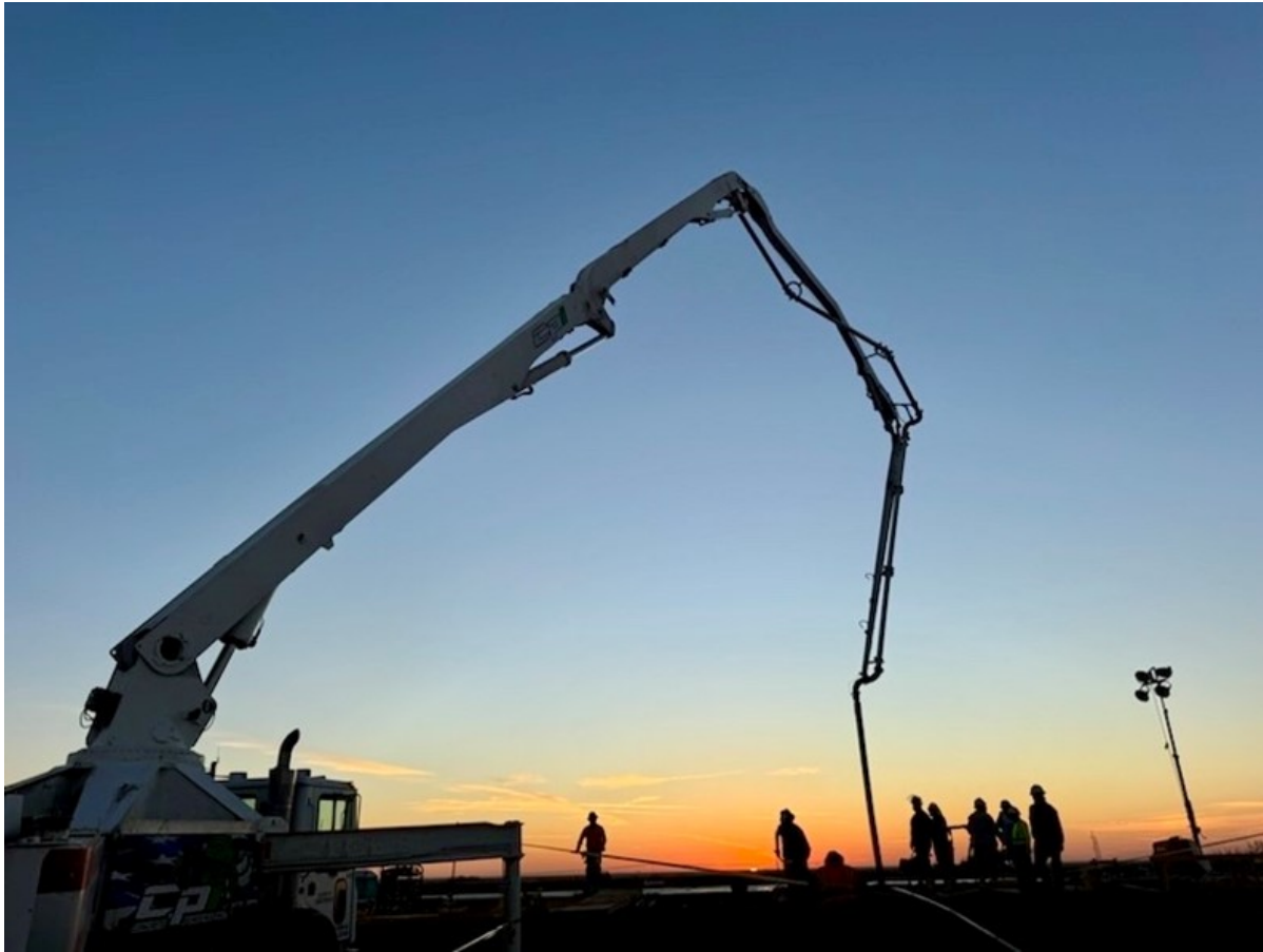
Laying concrete for one of the miner wings at Black Pearl
