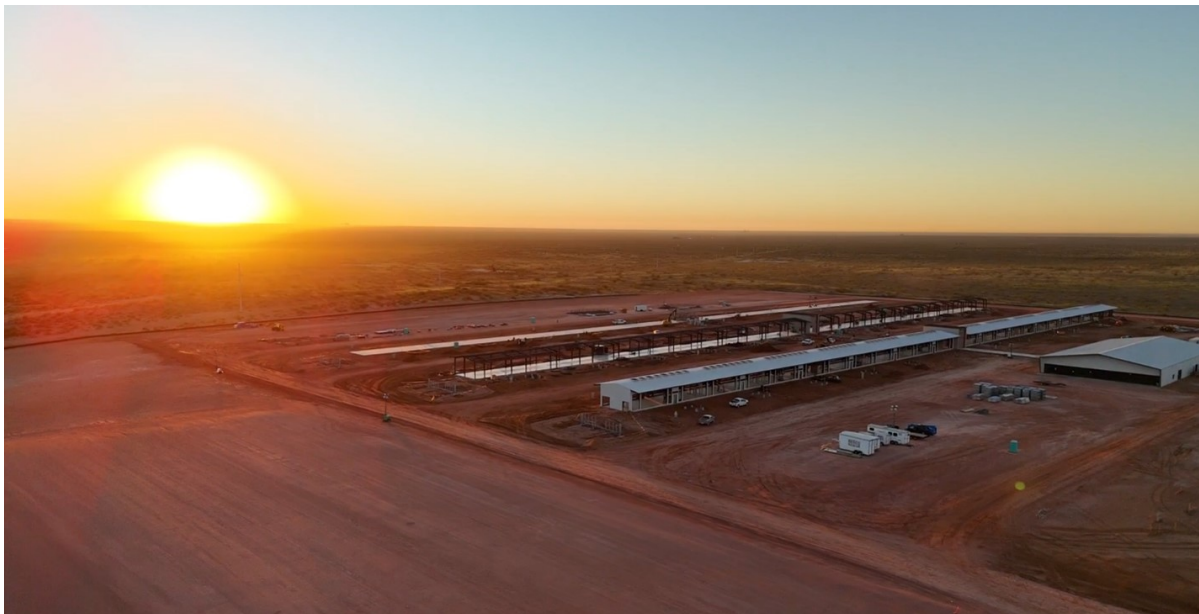
Construction at Black Pearl Site
