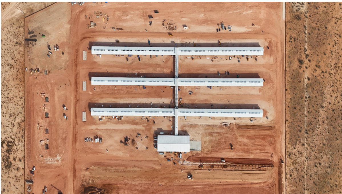
Construction at Black Pearl site
