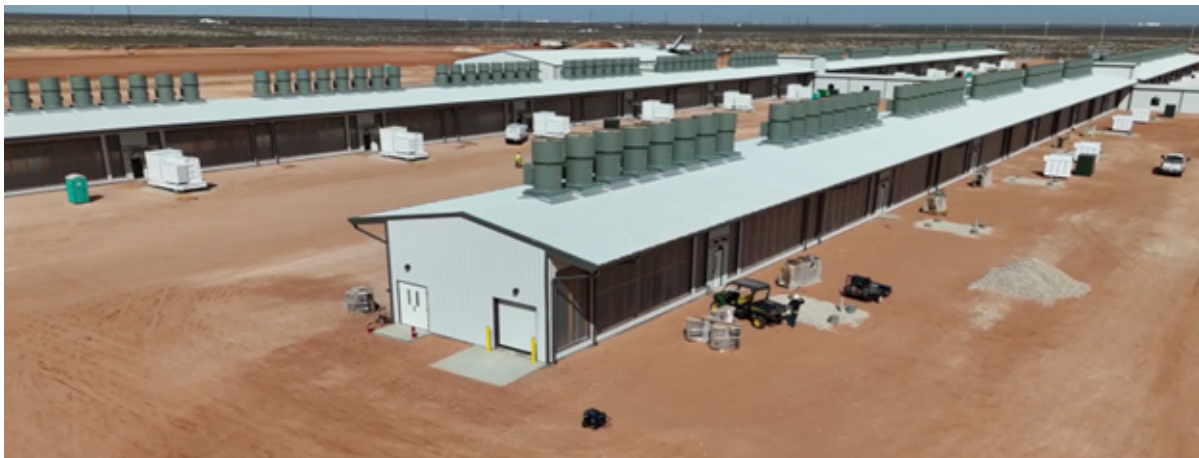
Black Pearl construction continues to progress ahead of schedule.
